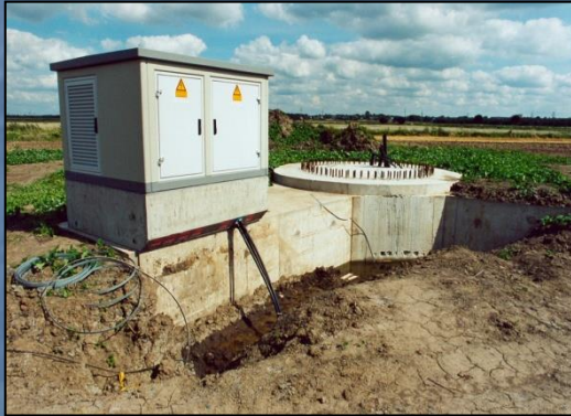
Foundation for a tubular tower to support a turbine. Note the positioning frame to ensure alignment of the tower flange.
