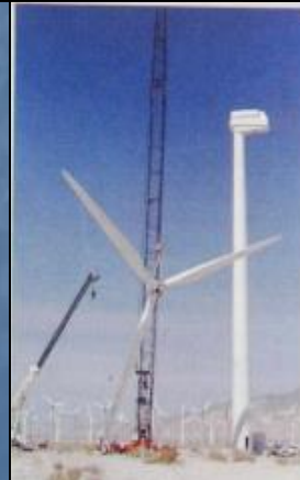
Assembling the rotor. Note the
