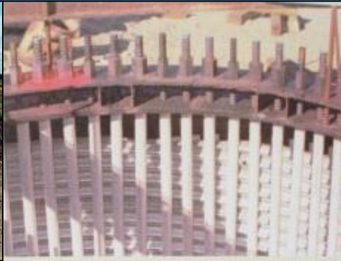
Threaded rebar used for tensioning of the rebar. Unlike traditional system of the excavation is only partially filled with concrete.
