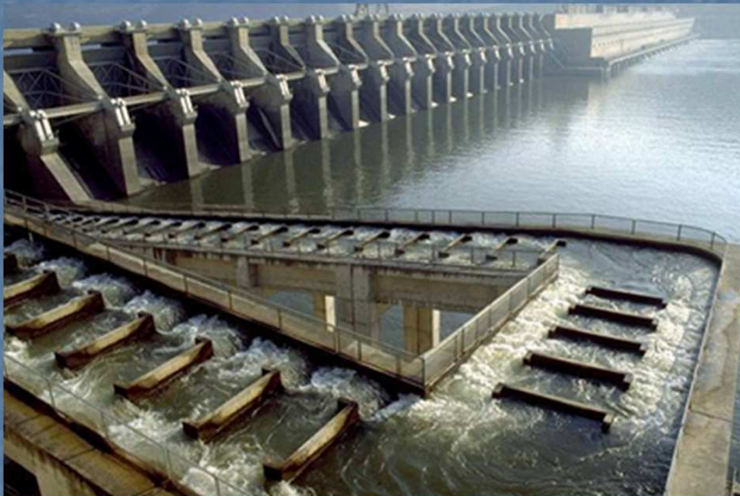
John Day Dam fish ladder on the Columbia River
